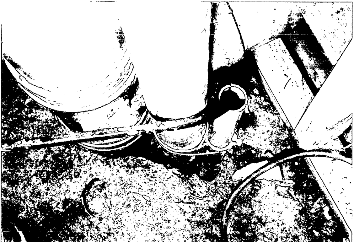
Figure 2. Service cupboard showing gaps between pipes and concrete and conduit taking cable.
