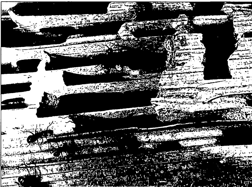
Figure 2. Carpenter ant infestation showing galleries and runways.
