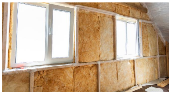
Figure 4: Example of a green-construction house built with sheep wool.
