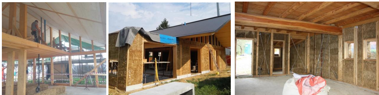
Figure 1-2-3: Example of straw-insulated in green-building.
